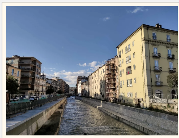
The river Sabato, along whose banks Atripalda stands.
