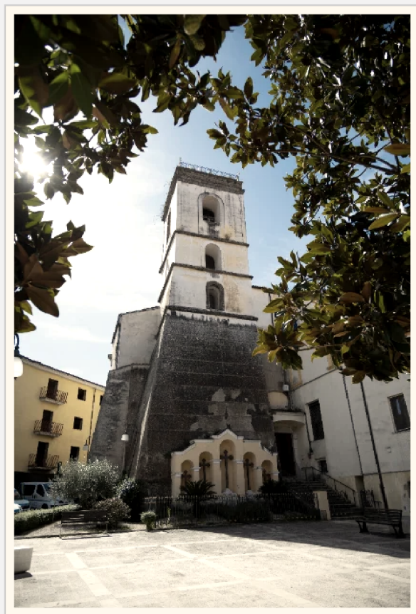
The bell tower of San Lorenzo, with its characteristic open gable profile.
